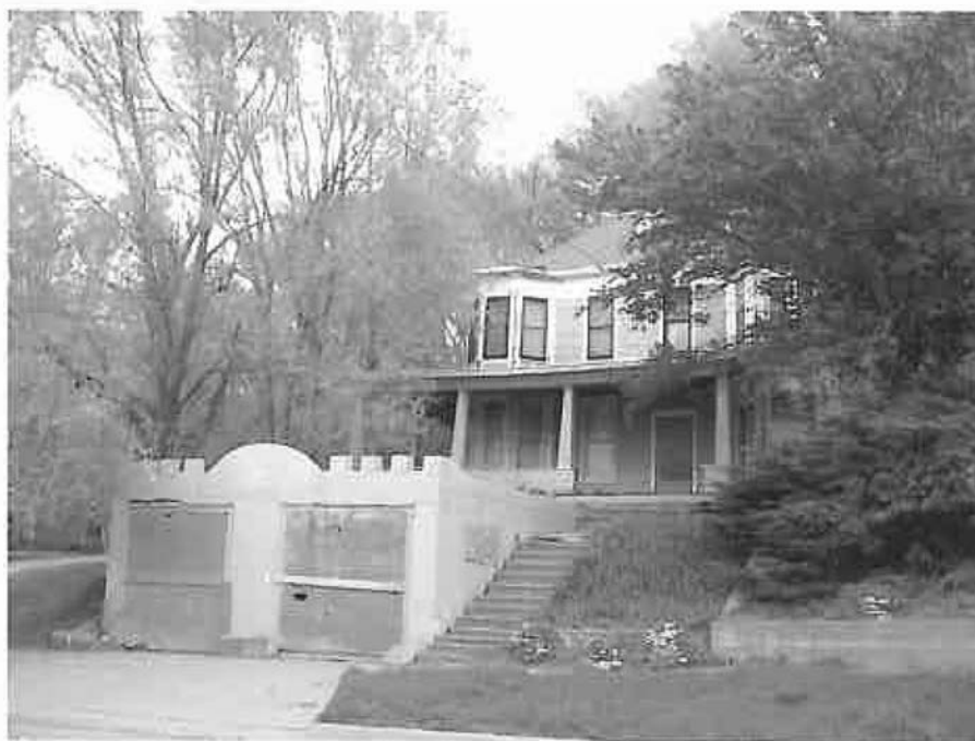
431 Park Avenue, Queen Anne/Stick style, with concrete garage inset in front slope Photograph taken by Tallgrass Historians L.C., 2008
