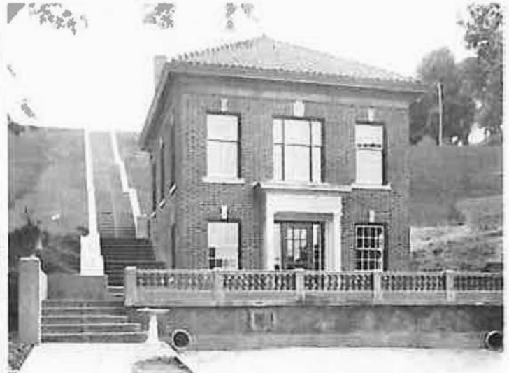
1930 photograph of the Glendale Pumping Station Note stairs (non-extant) going uphill to the reservoir
